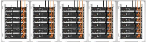
Make sure all dip switch of master batteries are R0XX, then turn ON batteries.
